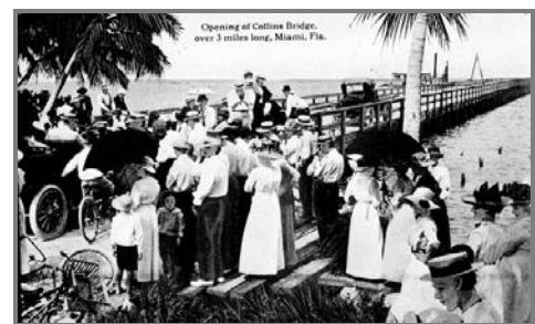
Collins Bridge was considered the "longest wooden bridge in the world." (Photo: Florida Photographic Collection)
